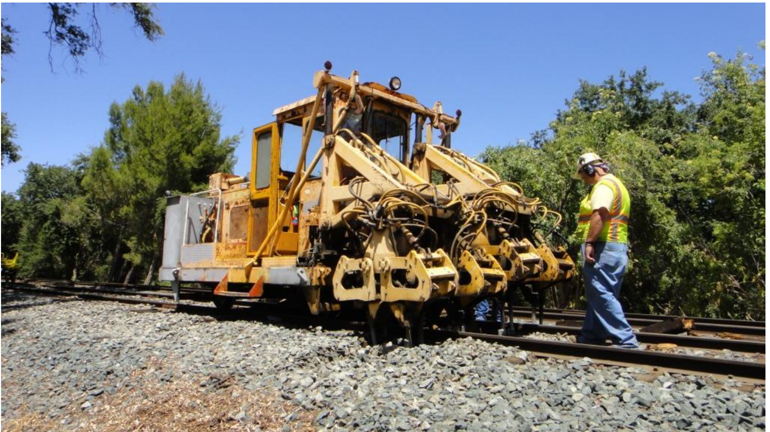
Meanwhile, further north, Mike F. guides Joe in the tamper as they tamp the ties installed last week
