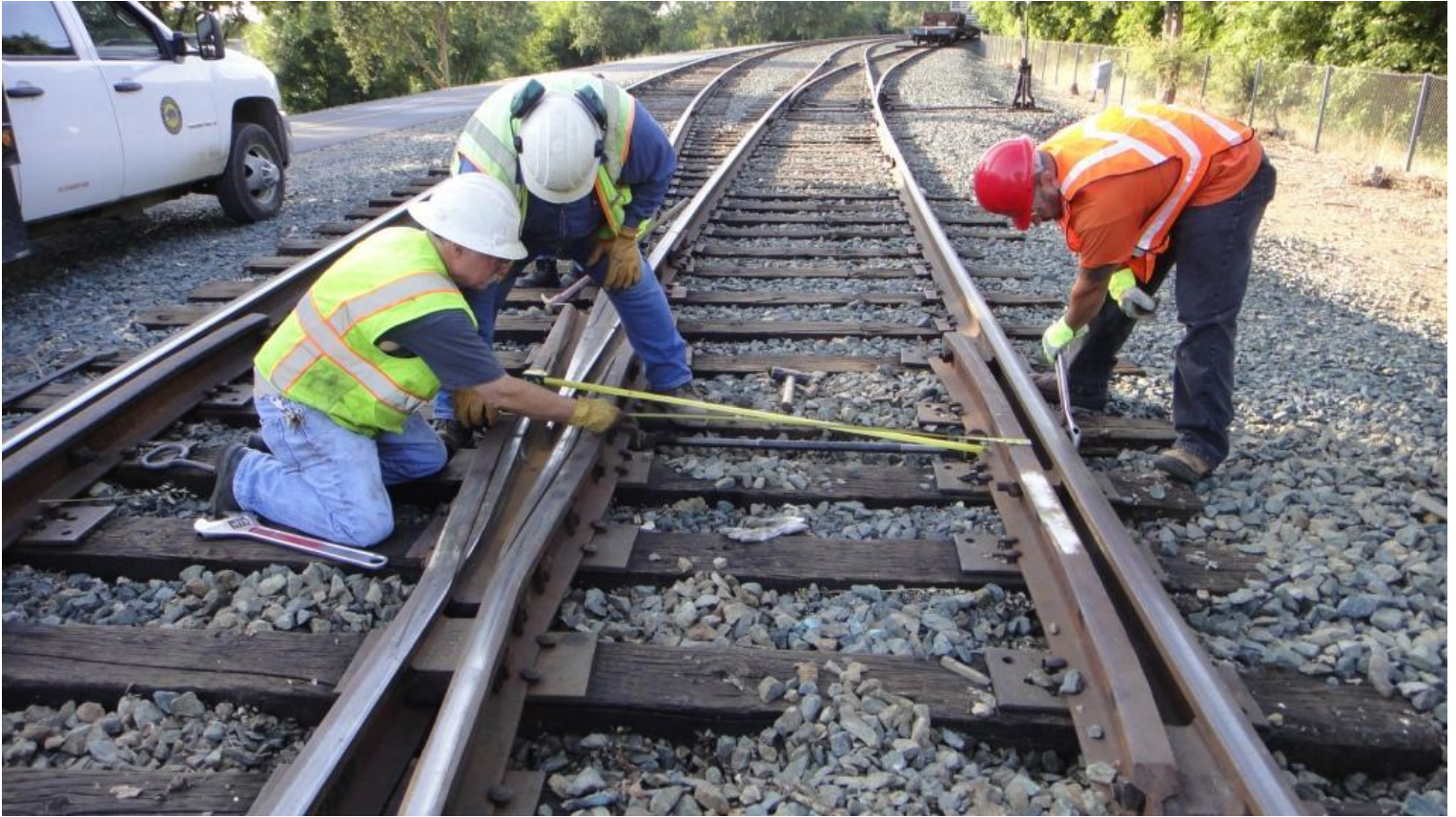
Mike H. and Frank measure guard-face and guard-check while Joe tightens down the gauge-rod
