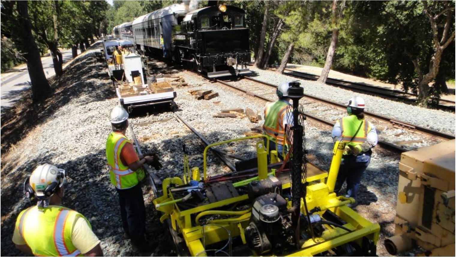
While deploying the rail-lifter, the crew is distracted by the appearance of the Granite Rock 10 – and who can blame them?
