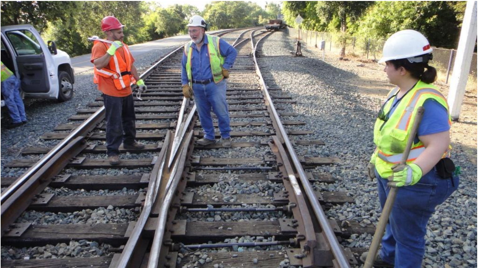
The Team surveys the successful installation of three gauge-rods at the frog of Switch 20
