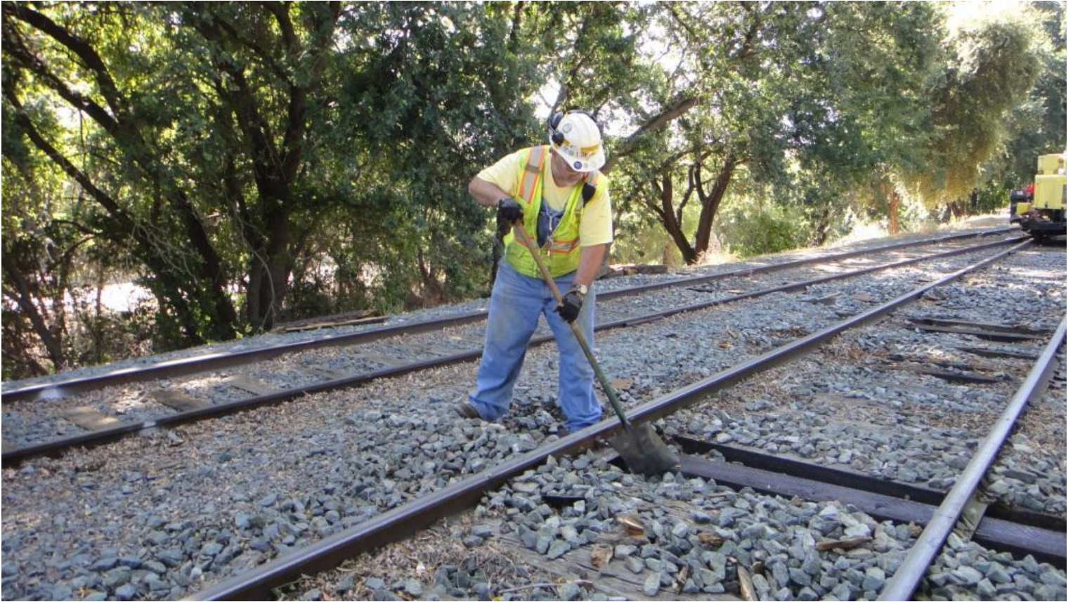
Dig, dig, dig! Mike F. fills in the crib with rock around a newly inserted tie
