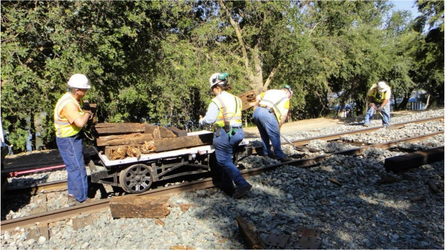
John and Heather load tie debris on a flat-car while Frank and Mike F. shift rock into the cribs of newly inserted ties
