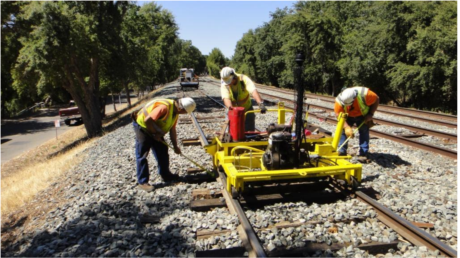
Mike F. operates the rail-lifter so that John and Frank insert tie-plates between the base of the rails and the ties
