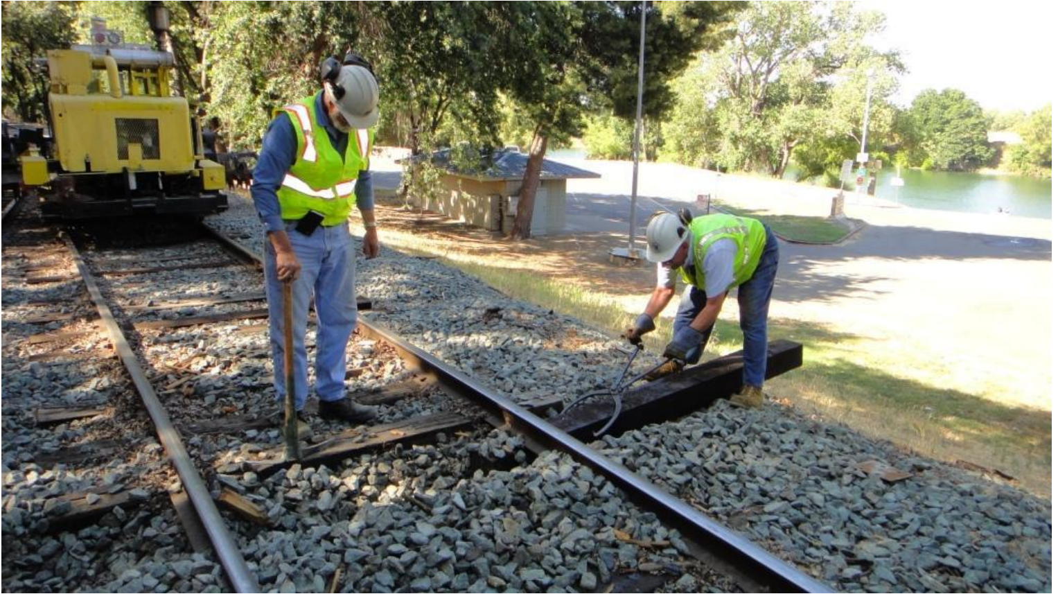
Clem and Alan pull out half-installed tie went in catawampus and jammed last week
