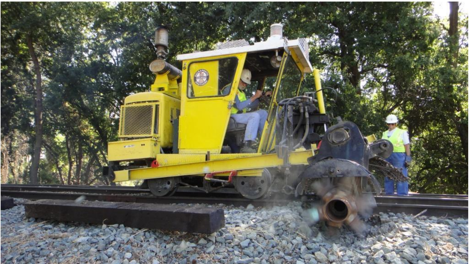
With the tie removed, Alan in the scarifier/insertor digs a more level crib
